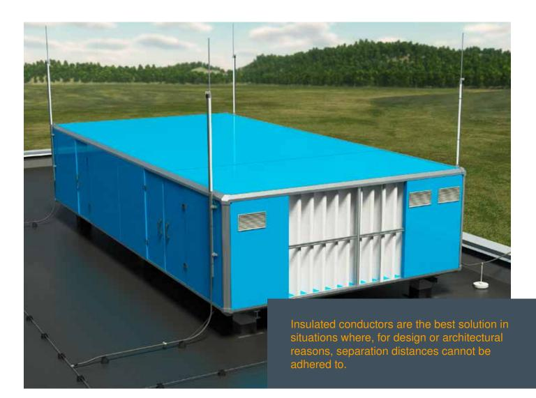
isCon<sup>®</sup> can safely master air separation distances of 0.75 m – in accordance with VDE 0185-305-3 (IEC 62305-3)
